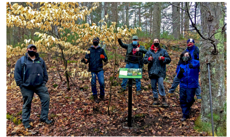
Connor Jewson (third from left) and fellow scouts install an interpretive sign with Land Steward Owen Grey (far left).
