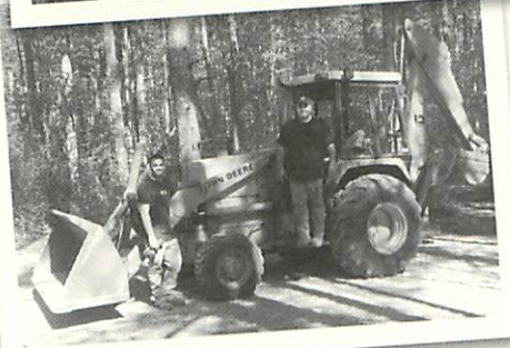
Trailblazers volunteers (top) at Halfway Pond in Plymouth and (below) installing the parking area at the Delano property in Rochester.
