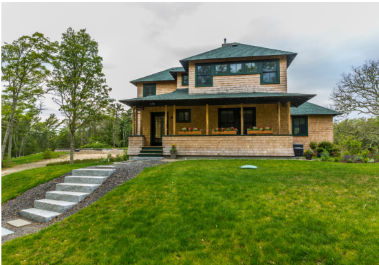
Wildlands' newly renovated office in Plymouth with the foundation of the Community Conservation Barn in the background (2014).
